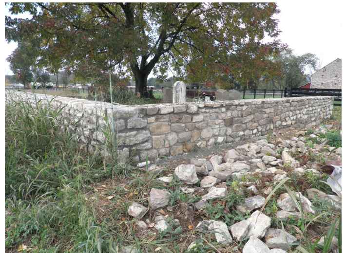
Two completed walls BCAGP restored on the DeTurck 2 Burial Ground.
