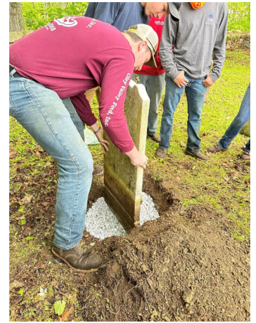
Jacob completing a stone repair in Bieber Leshner.
