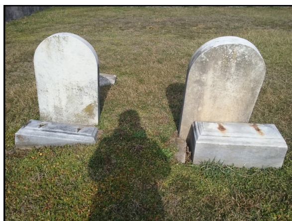
Above: Curved headstones in the Herbein, Oley , have broken metal rods & are off their bases.
