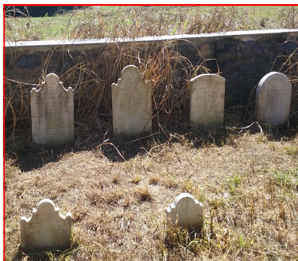
Above: Curved headstones in the Herbein, Oley , have broken metal rods & are off their bases.
