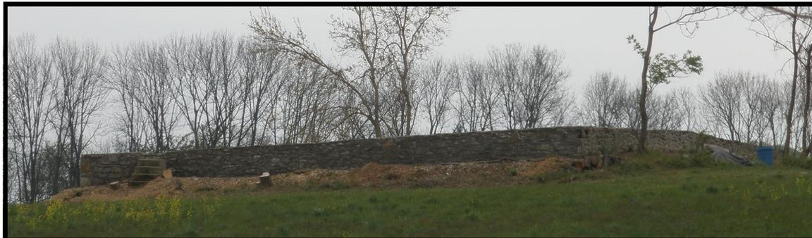
Left: front view after trees were removed and shredded and the front wall was repaired and re pointed.
