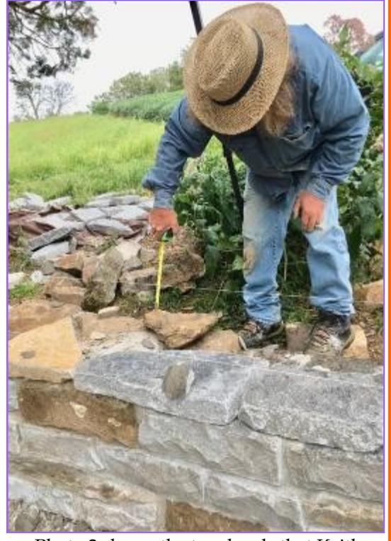
Photo 2 shows the two levels that Keith had to engineer to stabilize the wall
