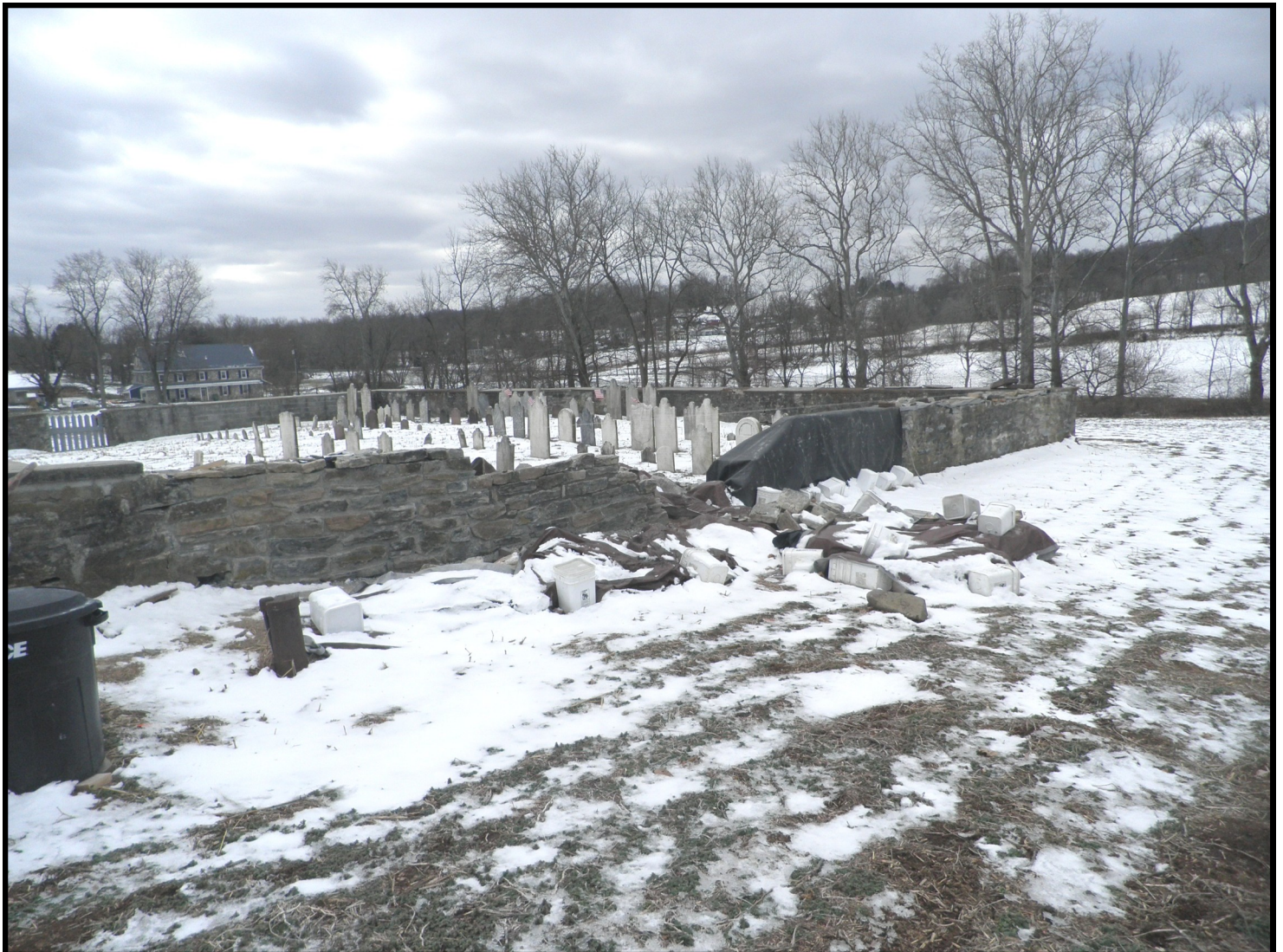
The entire rear wall is being repaired and re pointed
