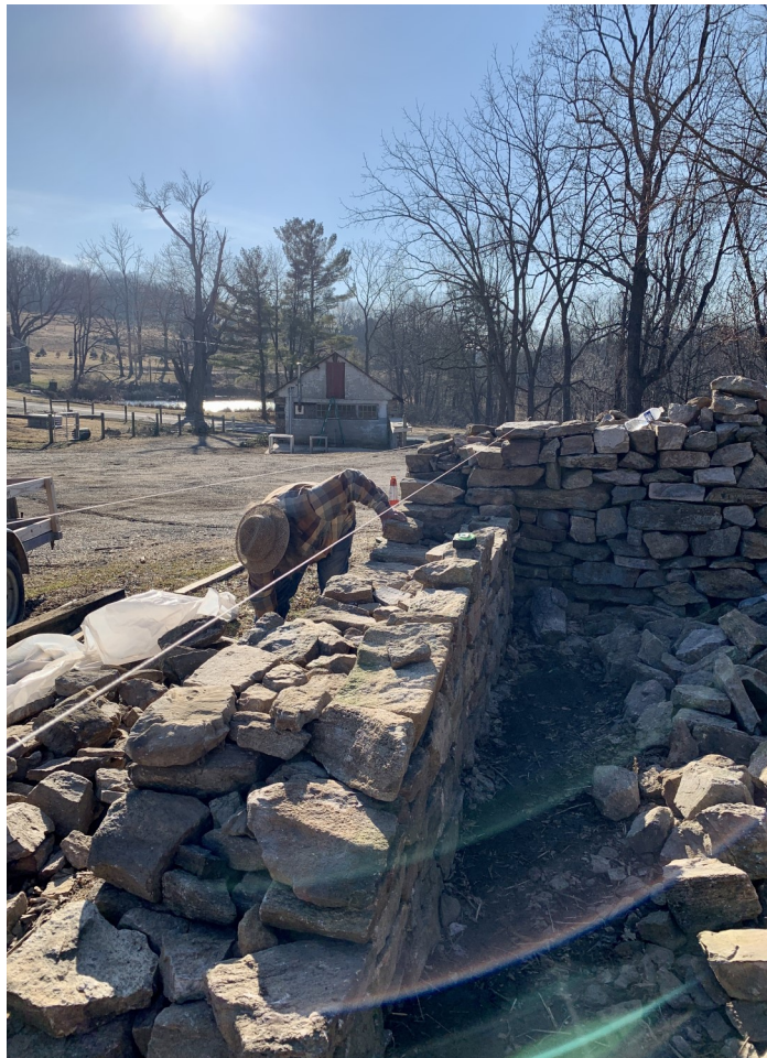
Keith busy at work rebuilding the wall surrounding the Conrad Burial Ground in Rockhill Township and resetting a stone that was previously buried (more photos on page 8)
