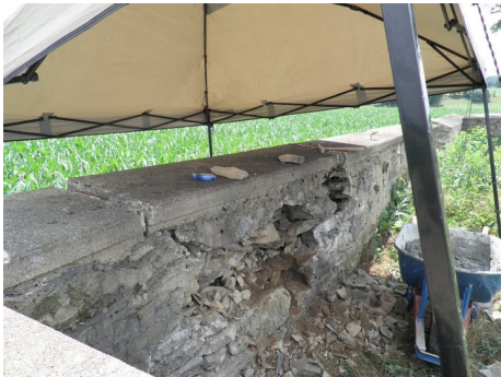
An example of the deterioration can be seen (left), as well as a section of the wall that has been restored (right).
