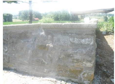
An example of the deterioration can be seen (left), as well as a section of the wall that has been restored (right).
