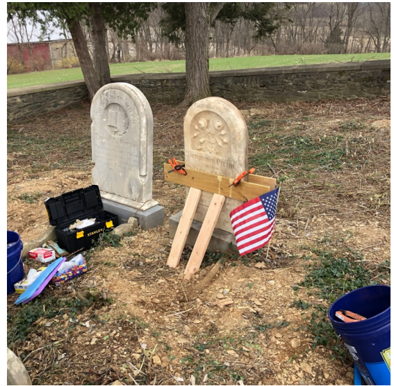
Repair work in progress April 3rd, 2022
