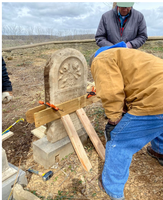
Repair work in progress April 3rd, 2022
