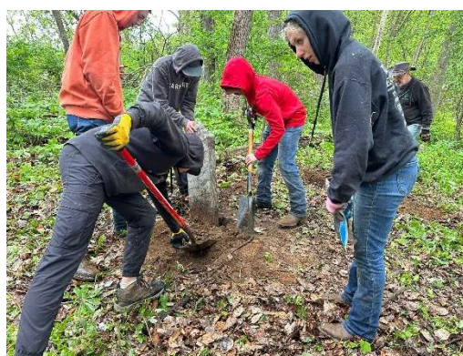
Stone Repair at Rauch
